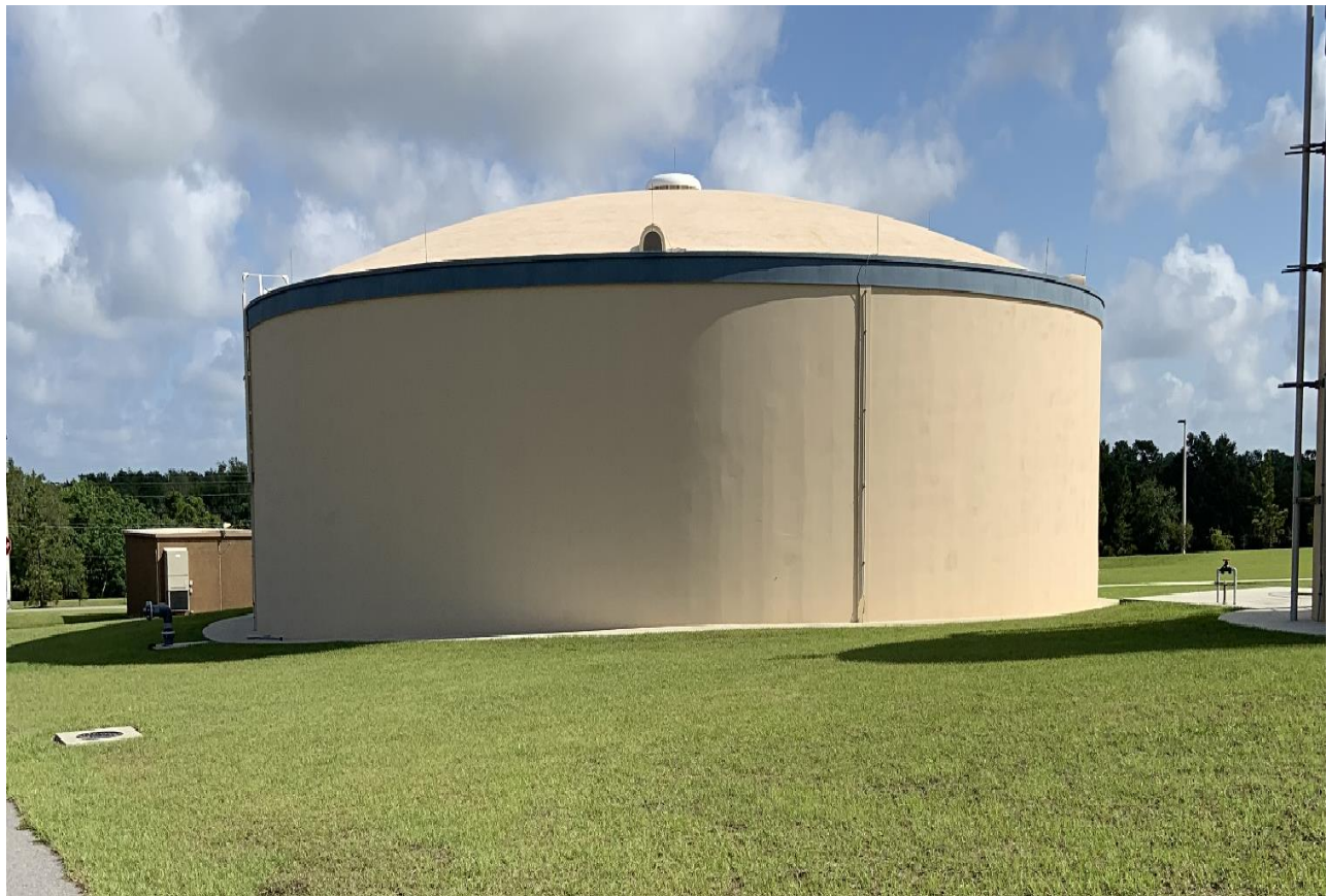
Figure 1 Central Regional Water Production Facility
