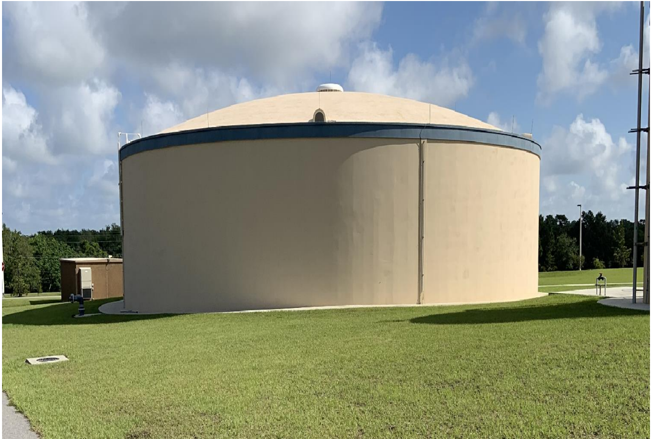
Figure 1 Central Regional Water Production Facility
