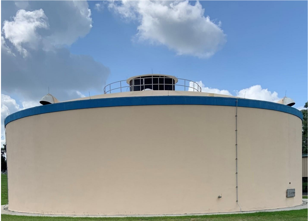
Figure 1 Cherry Hill Water Treatment Facility.
