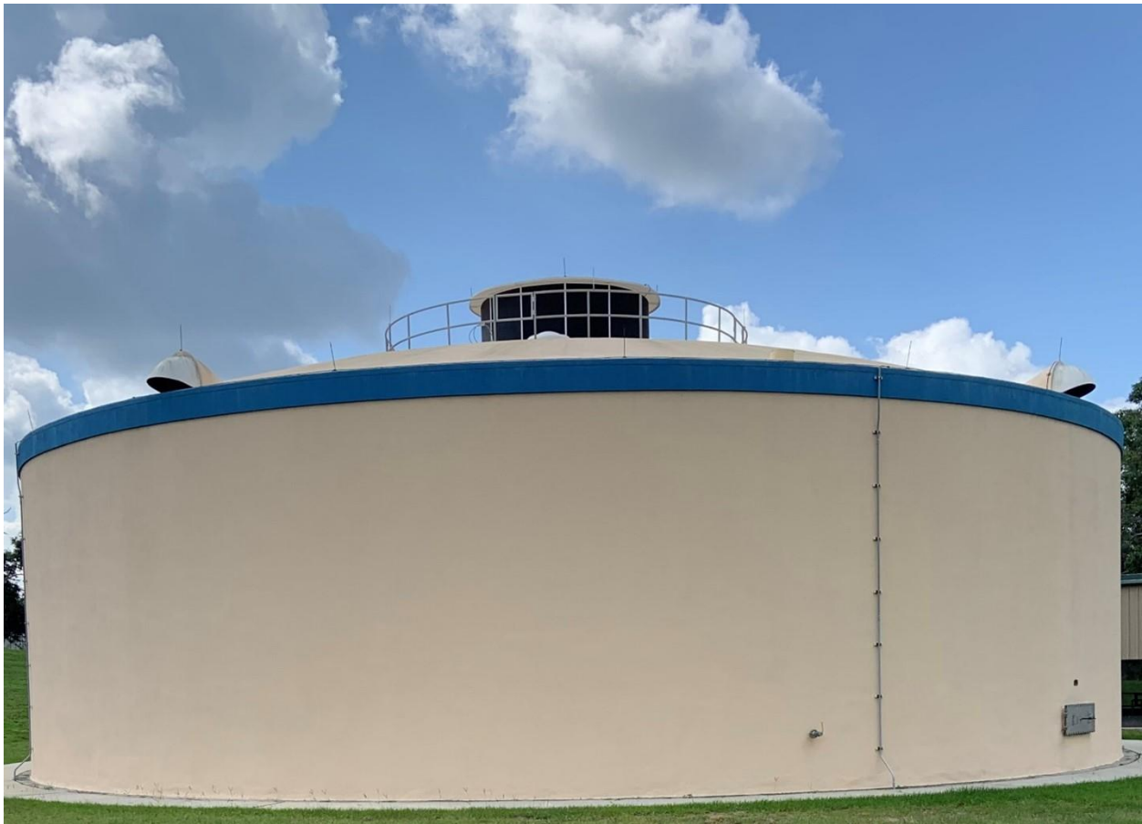
Figure 1 Cherry Hill Water Treatment Facility.
