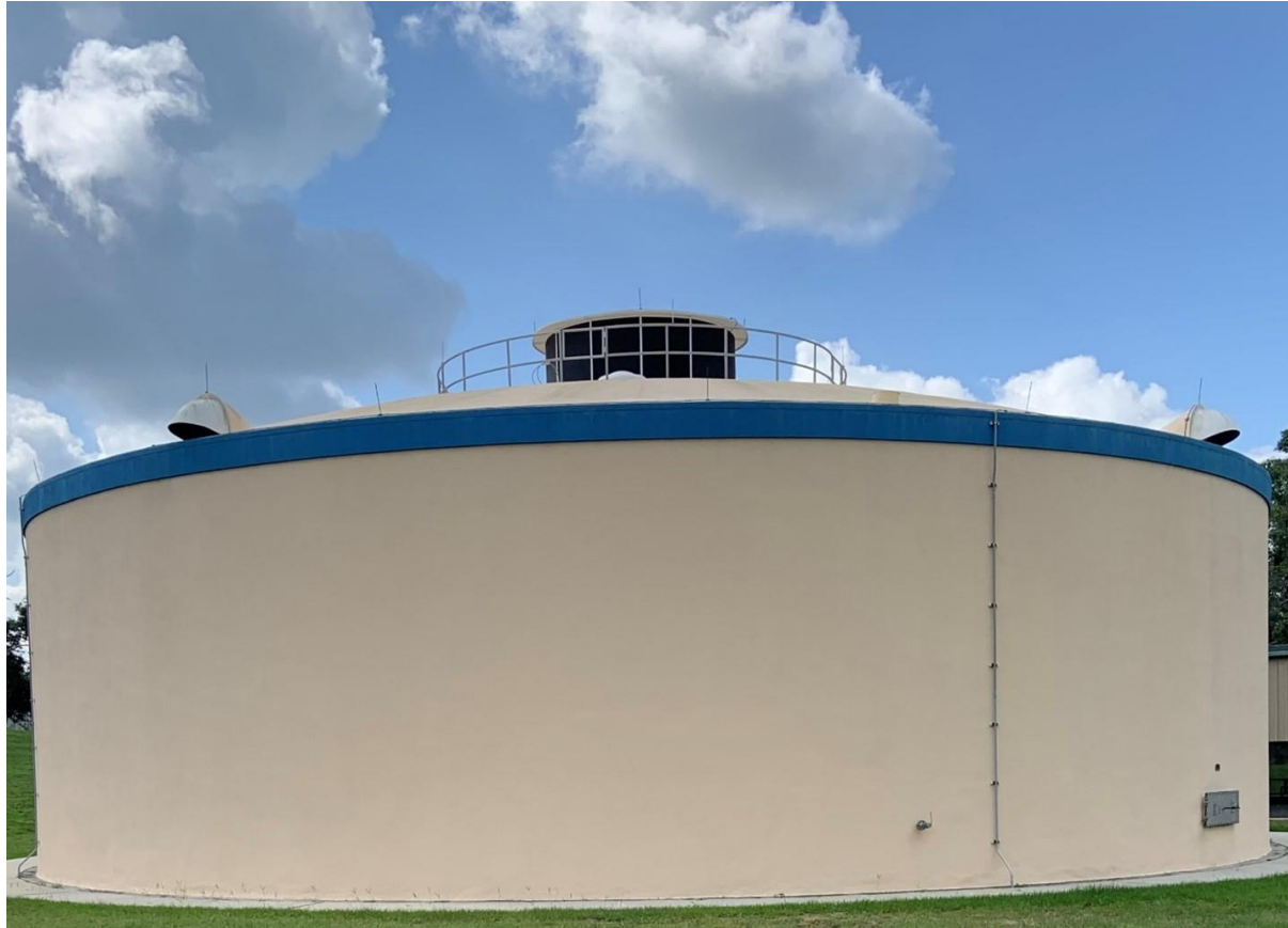
Figure 1 Cherry Hill Water Treatment Facility.
