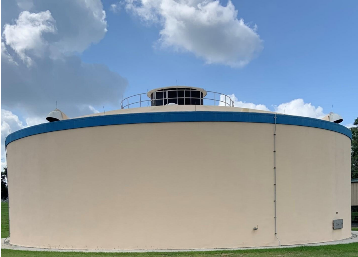
Figure 1 Cherry Hill Water Treatment Facility.
