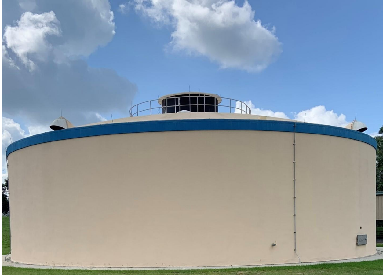
Figure 1 Cherry Hill Water Treatment Facility.
