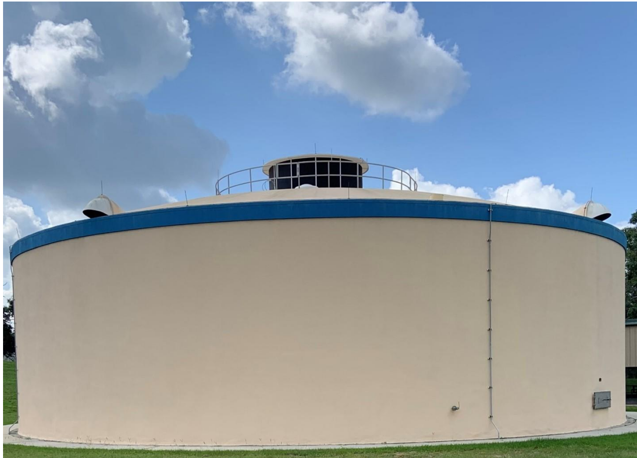
Figure 1 Cherry Hill Water Treatment Facility.
