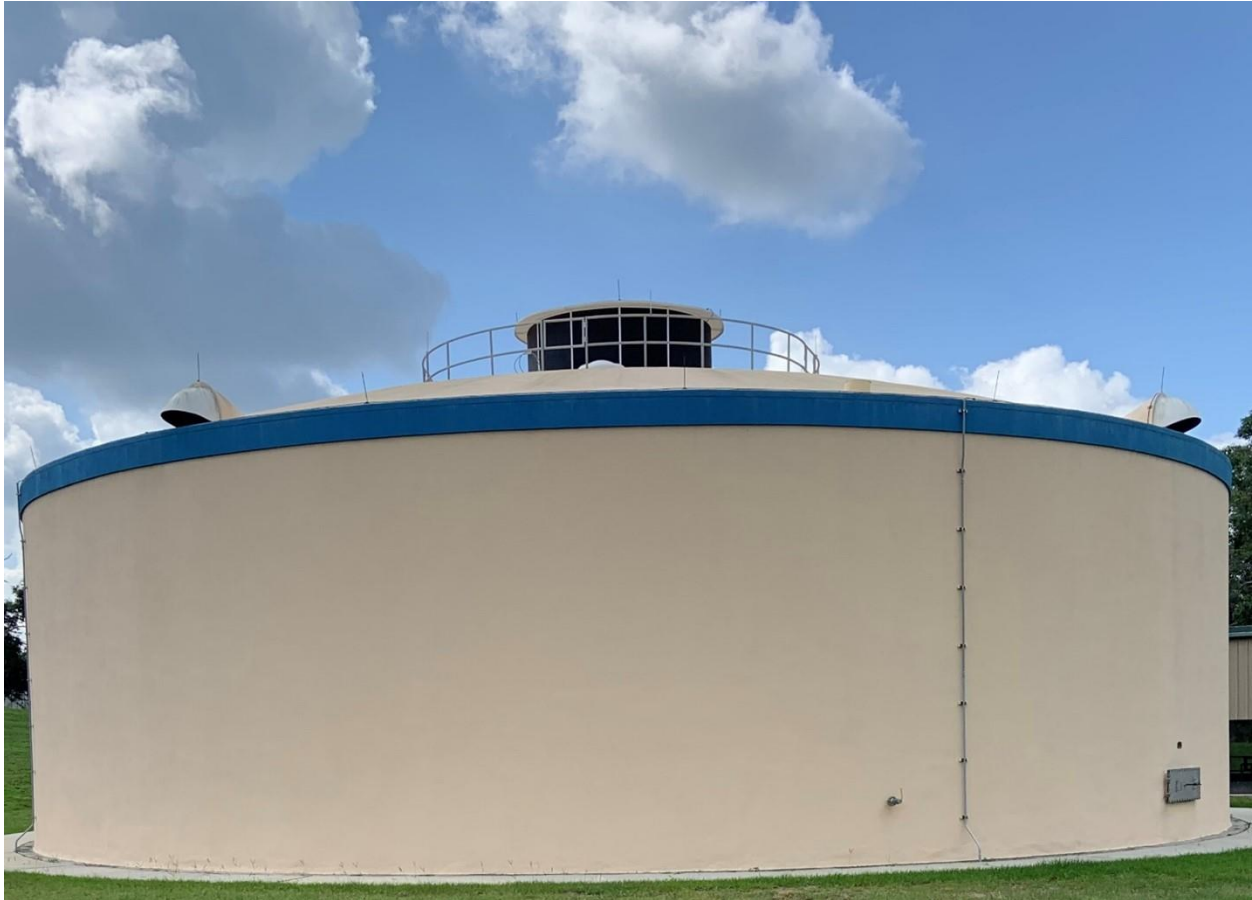
Figure 1 Cherry Hill Water Treatment Facility.
