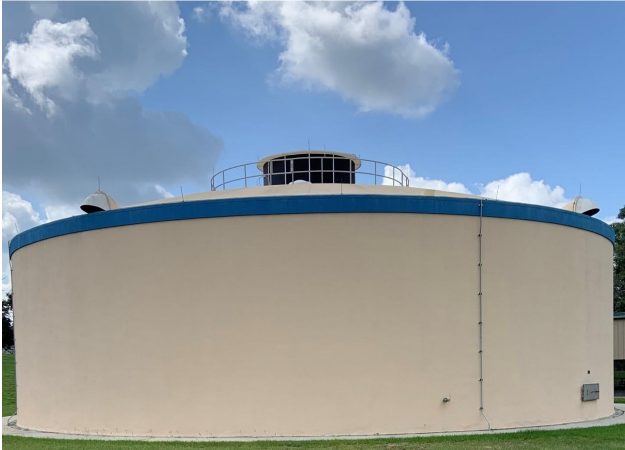
Figure 1 Cherry Hill Water Treatment Facility.
