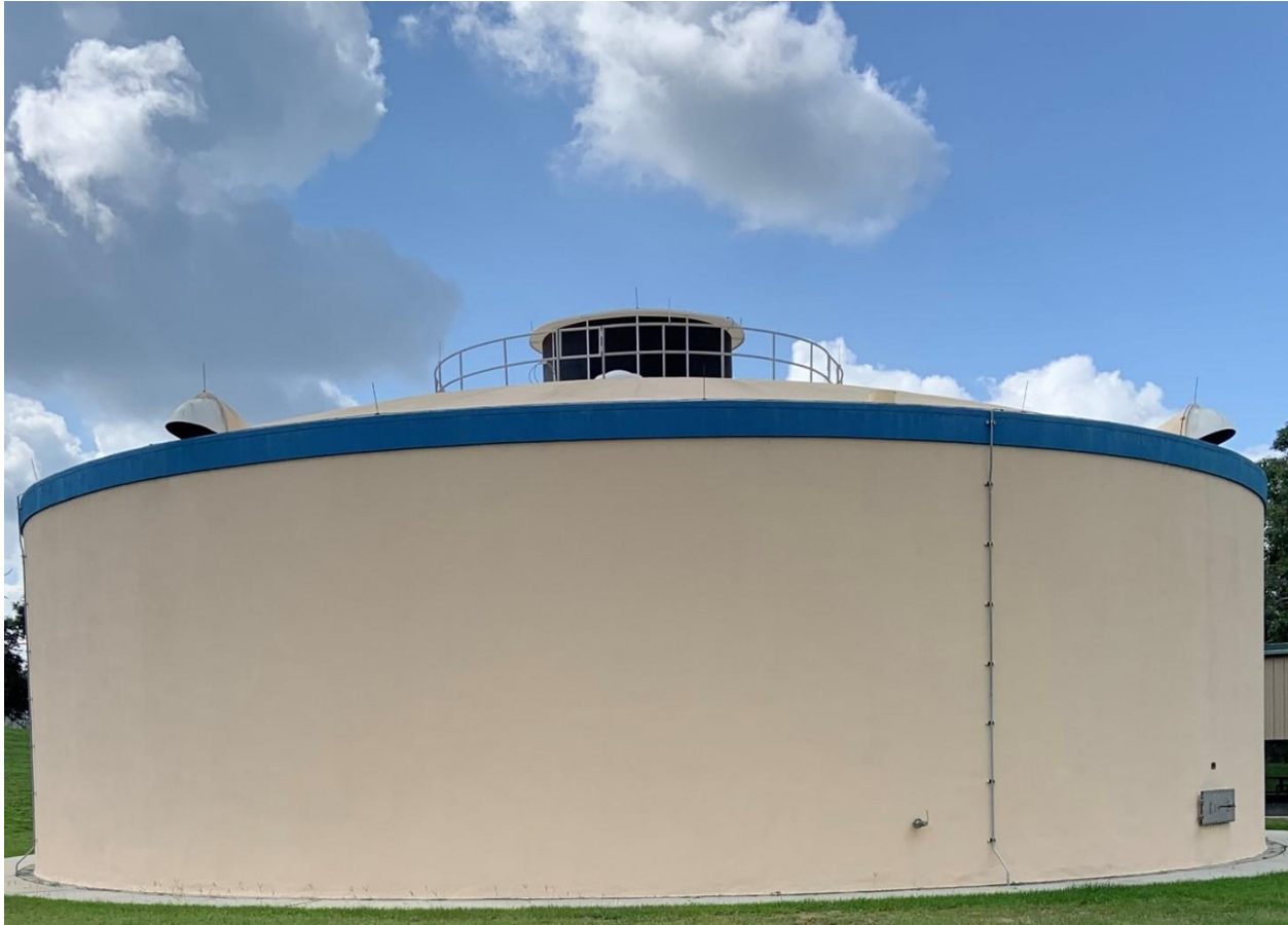
Figure 1 Cherry Hill Water Treatment Facility.
