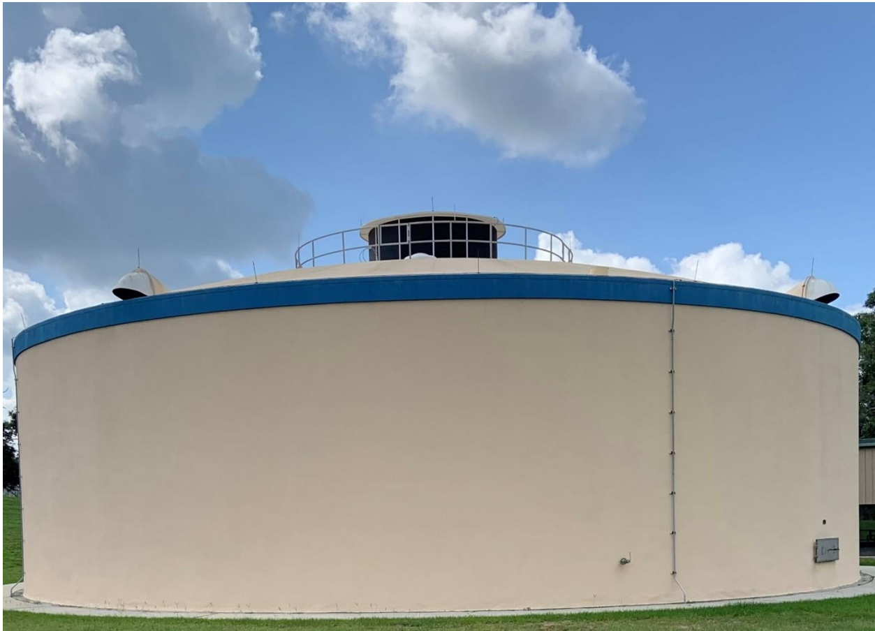
Figure 1 Cherry Hill Water Treatment Facility.
