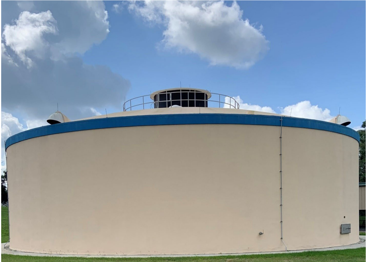
Figure 1 Cherry Hill Water Treatment Facility.
