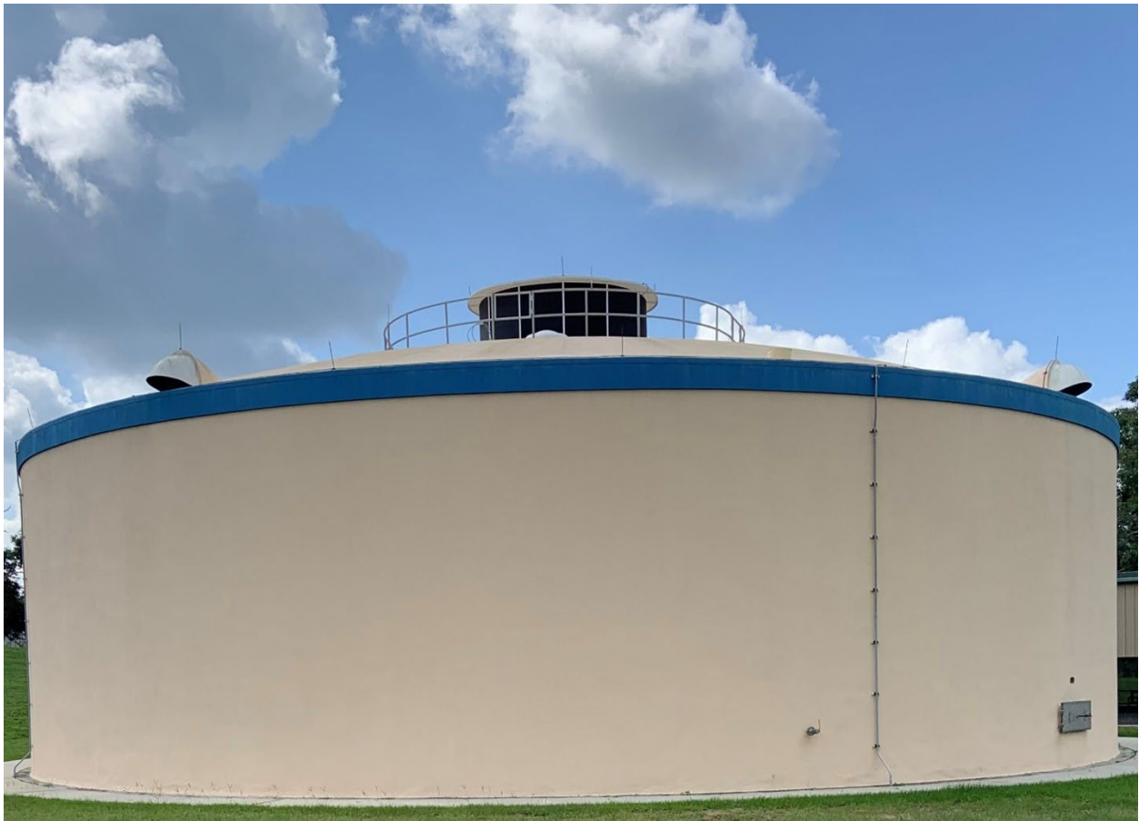
Figure 1 Cherry Hill Water Treatment Facility.
