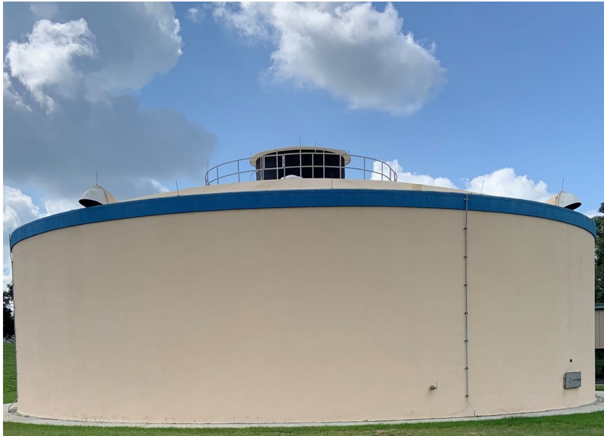
Figure 1 Cherry Hill Water Treatment Facility.
