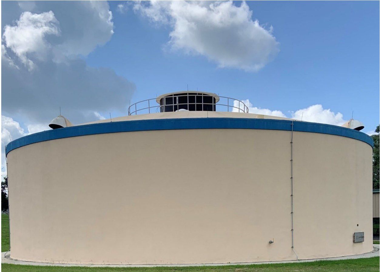
Figure 1 Cherry Hill Water Treatment Facility.
