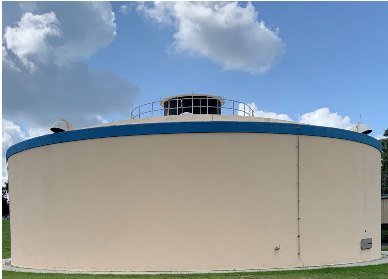
Figure 1 Cherry Hill Water Treatment Facility.
