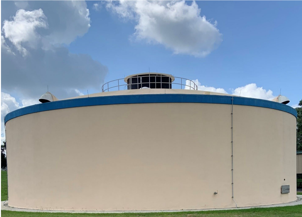
Figure 1 Cherry Hill Water Treatment Facility.
