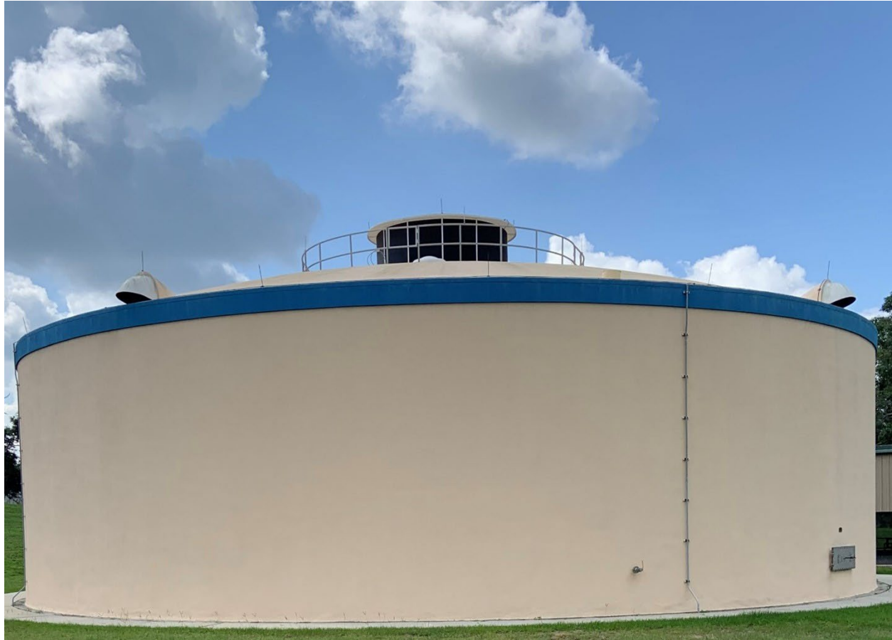
Figure 1 Cherry Hill Water Treatment Facility.
