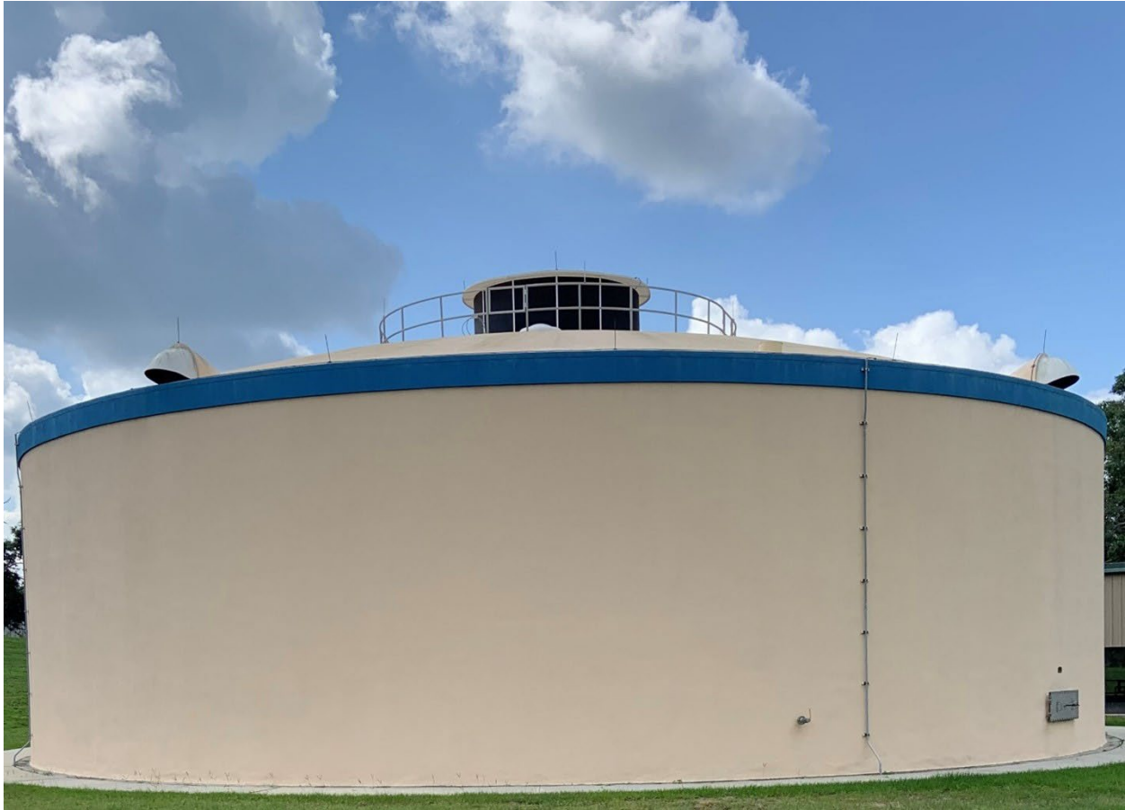
Figure 1 Cherry Hill Water Treatment Facility.
