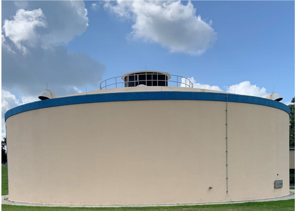
Figure 1 Cherry Hill Water Treatment Facility.
