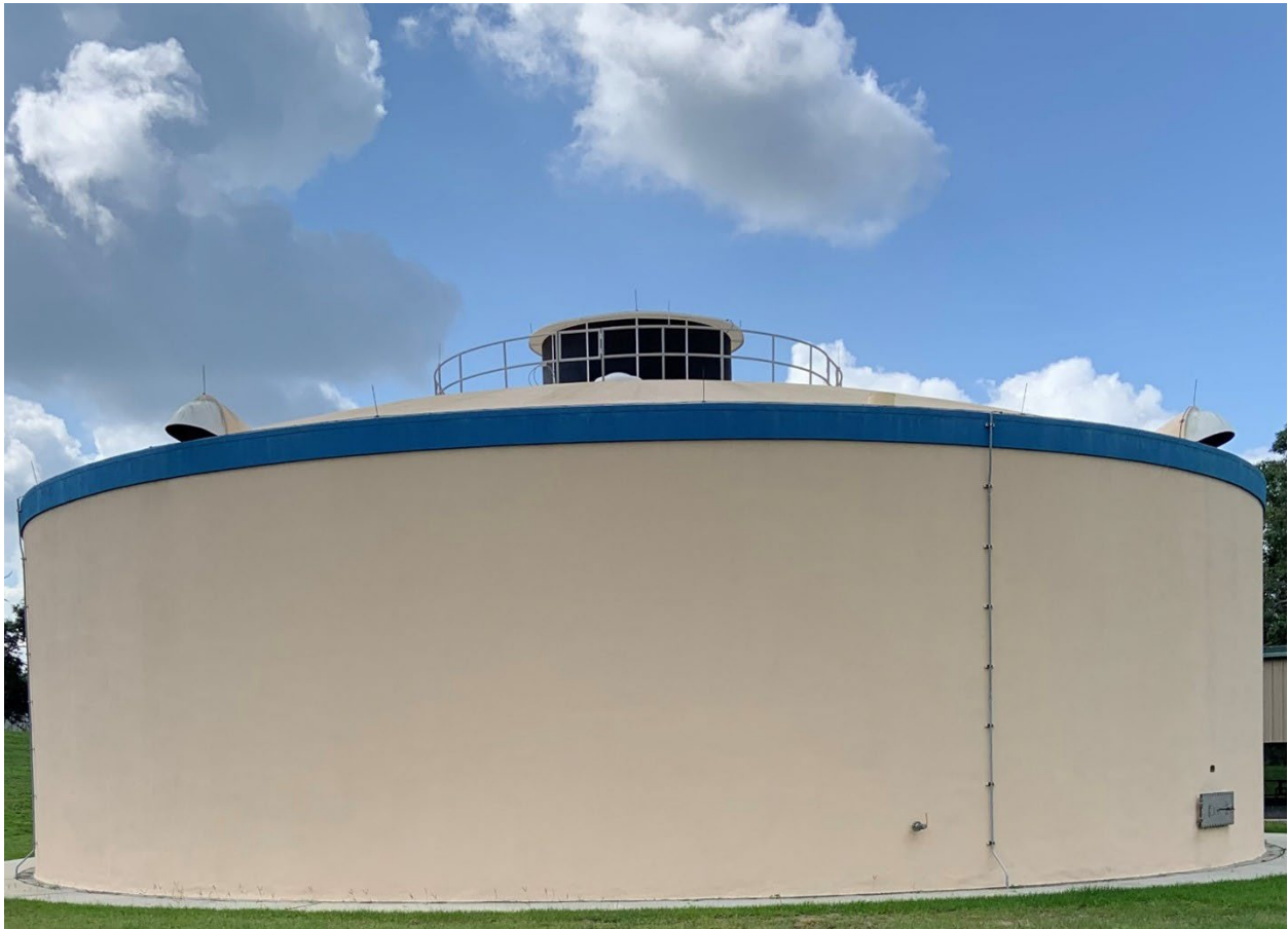
Figure 1 Cherry Hill Water Treatment Facility.
